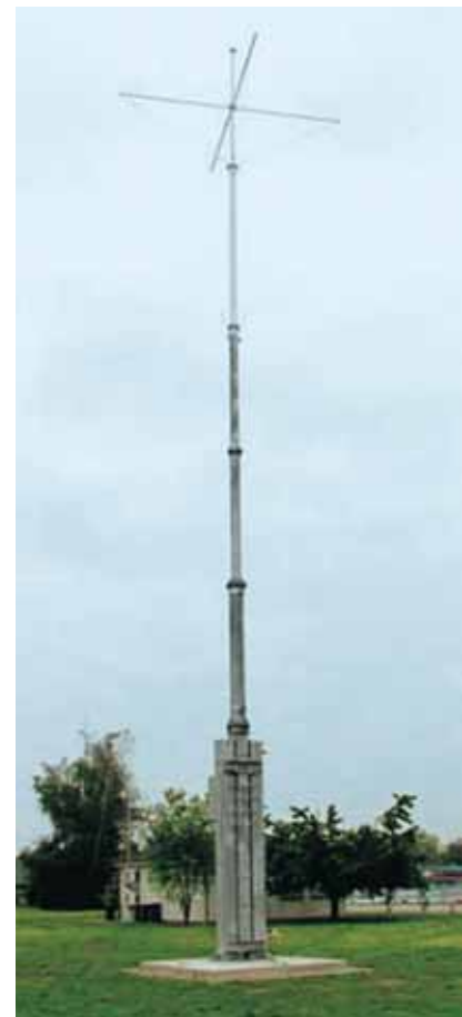
Abb. 4: Beacon-Sendemast in Iffezheim (293,5 MHz).
